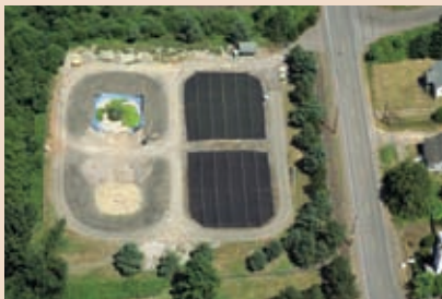
Boring Sewage Treatment Facility 13305 SE Richey Road Boring, OR 97009
