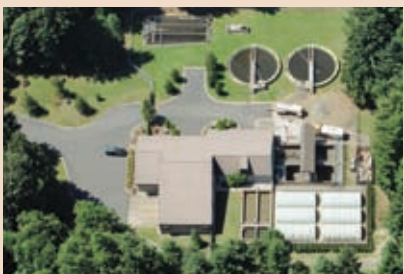
Hoodland Sewage Treatment Plant 24596 E Bright Ave. Welches, OR 97067
