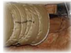
duct sealing and insulation
