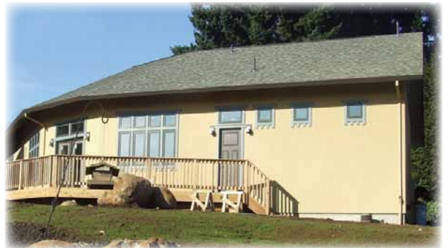
South facing windows allow the sun to warm the home in the winter while deeper-than-normal eaves prevent overheating in the summer.
