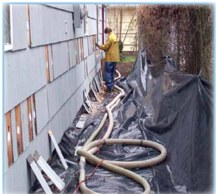
Contractor blows insulation into the walls of a home.
