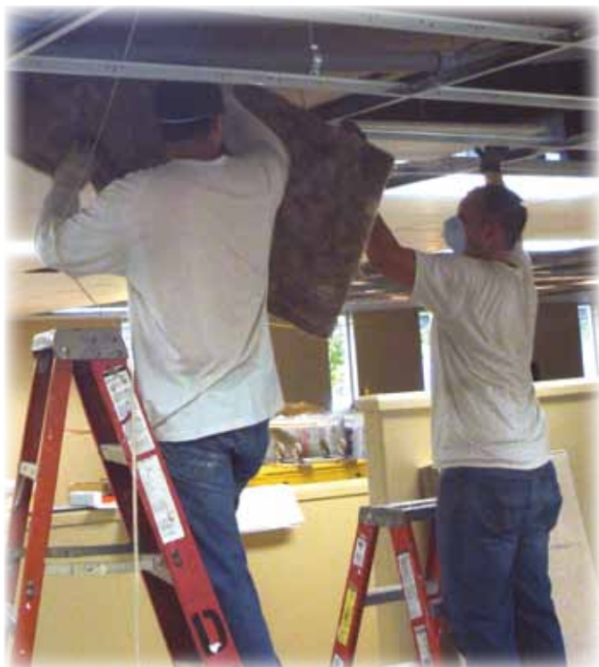
Installing ceiling insulation where none existed previously
